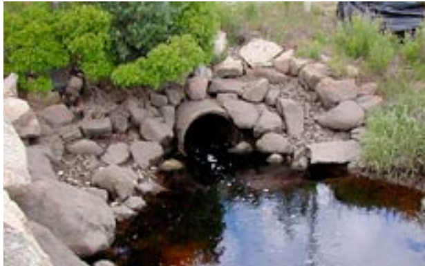
Old tidal restriction before replacement (MA CZM photo)
